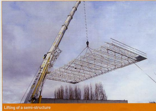
Lifting of a semi-structure
