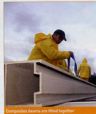
Composites beams are fitted together
